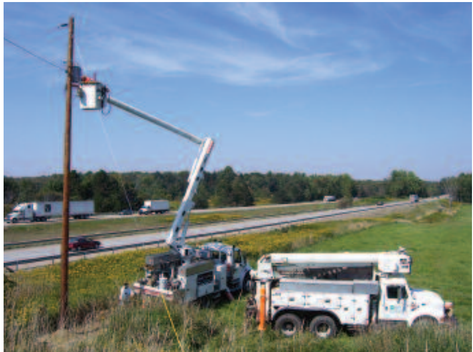
LINE WORK: Rebuilding an I-79 overhead line crossing.
