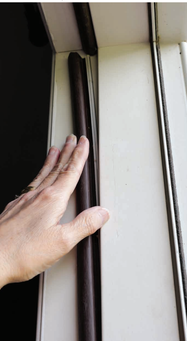
SEAL THE DEAL: Weather stripping helps seal drafts around exterior doors, which saves energy and improves comfort in your home.
