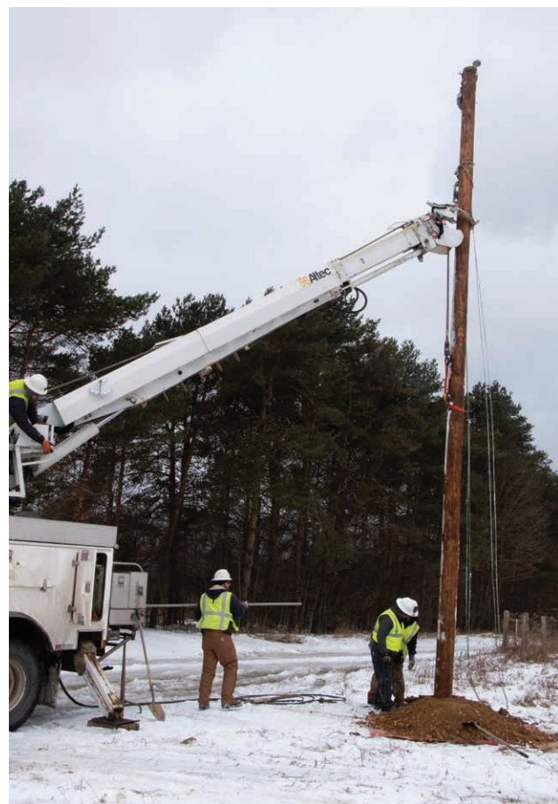
MAKING CONNECTIONS: United Electric Cooperative lineworkers set a pole for a new connection to a consumer-member in February 2019.
