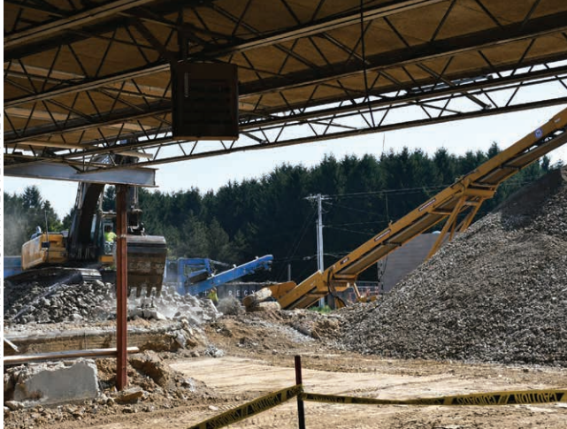
PROJECT BEGINS: Demolition of the old garage took place in May, June, and July, when walls, floors, and the concrete dock were knocked down. The concrete was ground up and will be used as fill for the new building, which will have a slightly larger footprint.
